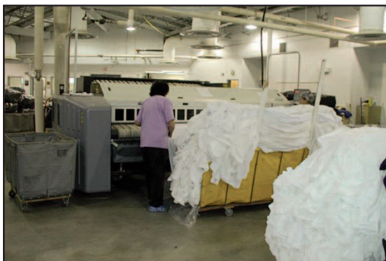
The facility finishes 8,000 sheets day using a Continental 32-inch, single roll flatwork ironer.
